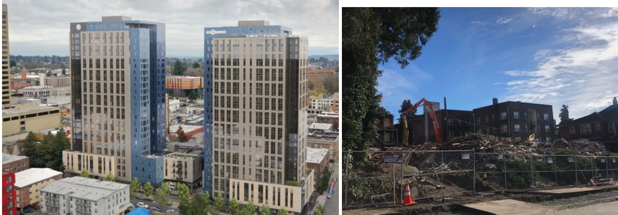
Above Left: A rendering of what the Standard towers will look like when finished. Above Right: Demolition of existing housing. Work as of Thursday, January 14.
