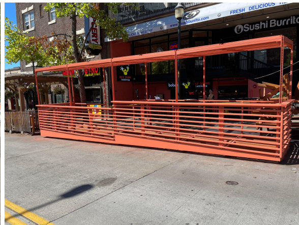
Construction of Boba Up's Outdoor Dining Structure
