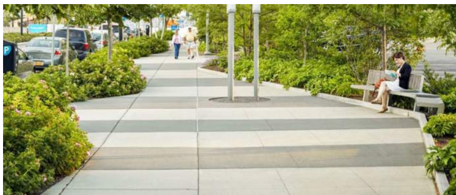
Topcast concrete examples of various finishes.
