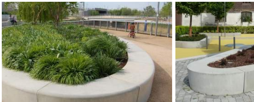
Raised precast concrete planters.
