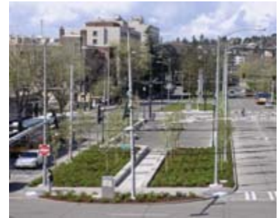
Figure 12. NE Campus Parkway Median
