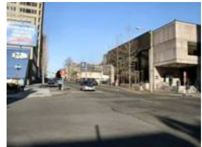
Figure 23. Northeast corner of NE 43 rd Street and Brooklyn Avenue NE.
