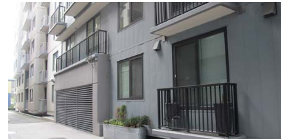
DC1-B1. The balcony and other design elements compatible with the façade have been integrated into the design of this parking garage.
