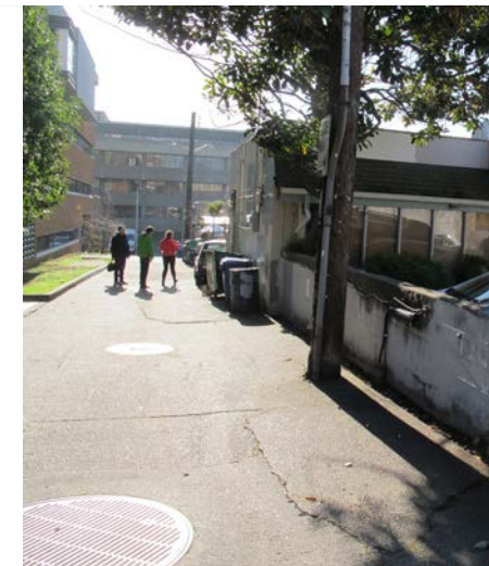
SCL utility pole and maintenance holes
