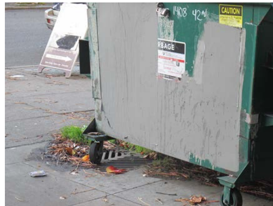
Catch basin at NE 43rd St (under dumpster) offset from alley centerline
