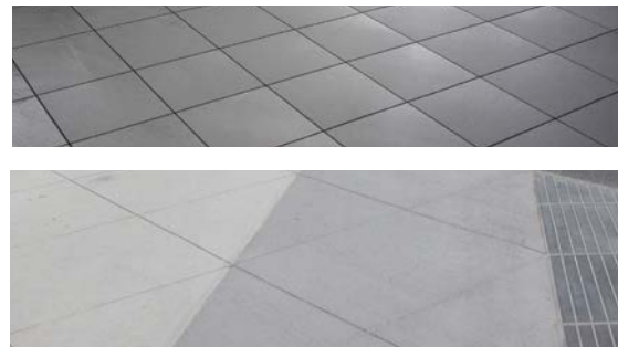
Examples of specialty concrete.
