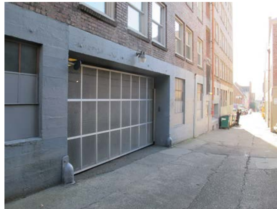
Malloy Apartments parking garage access
