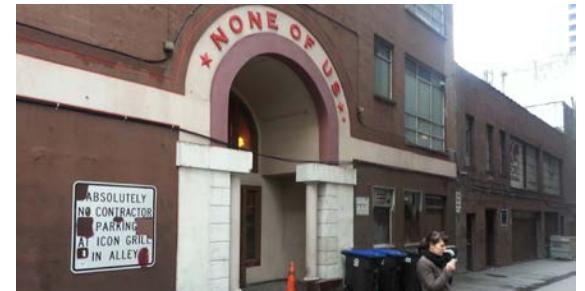
PL3-A2. Recessed entries distinguish an entryway but must be carefully designed for clear pedestrian visibility.
