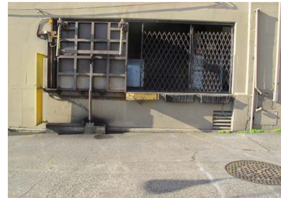
Maintenance hole near the University Bookstore loading dock
