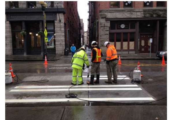
Nord Alley Zebra Crossing at Main St., Seattle, WA
