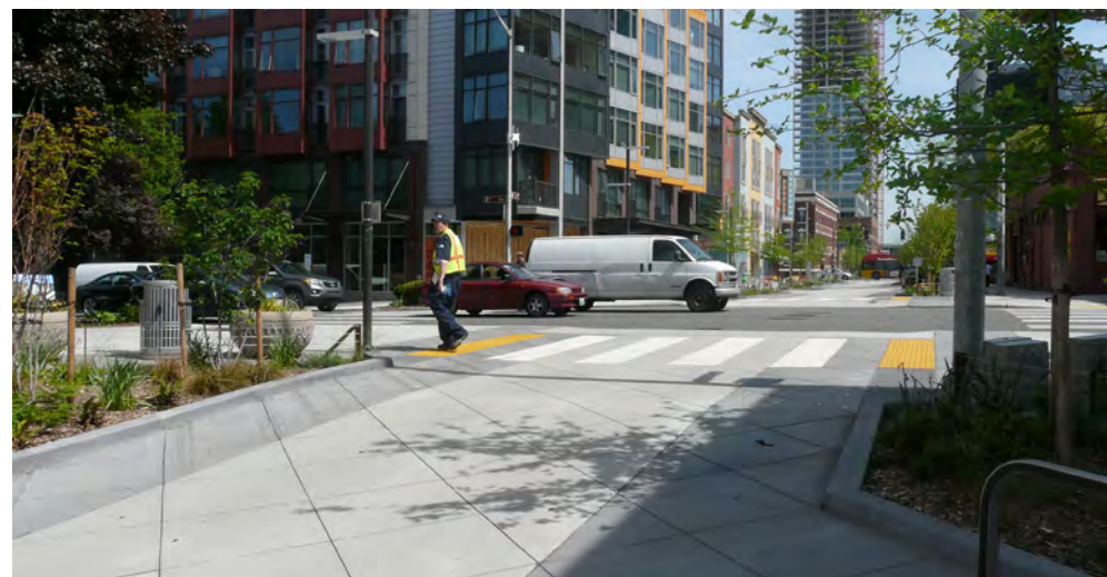
Thermoplastic paint should be used to clearly denote crosswalks.
