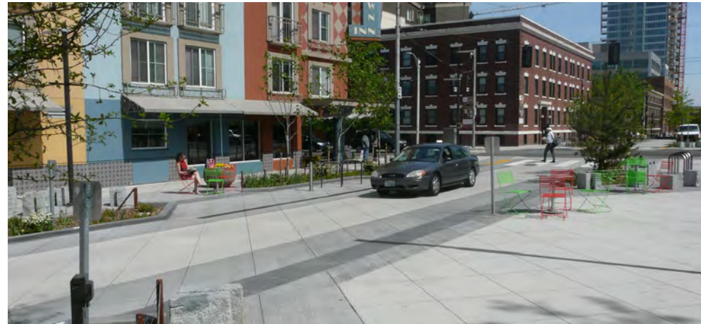
Bell St Park Boulevard is an excellent example of how zones of the right of way can be differentiated through changes in the concrete's texture, scoring and color.
